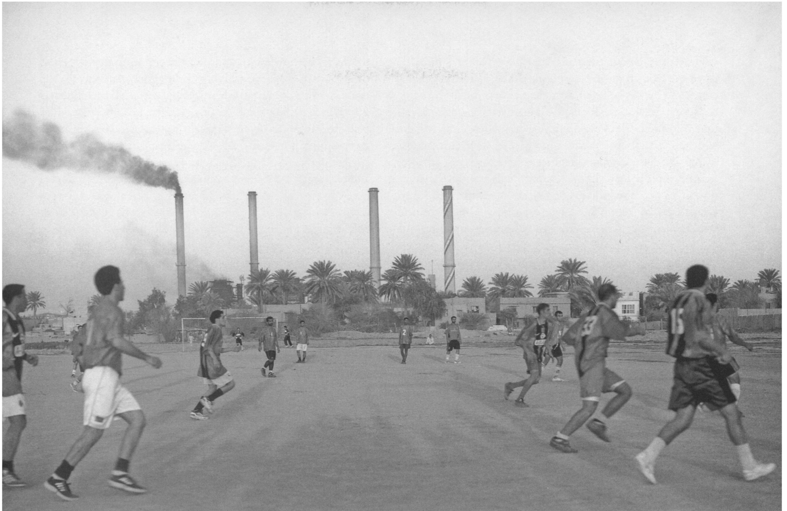
At Baghdad's Dawra power plant only one of four turbines function properly, April 2004.
